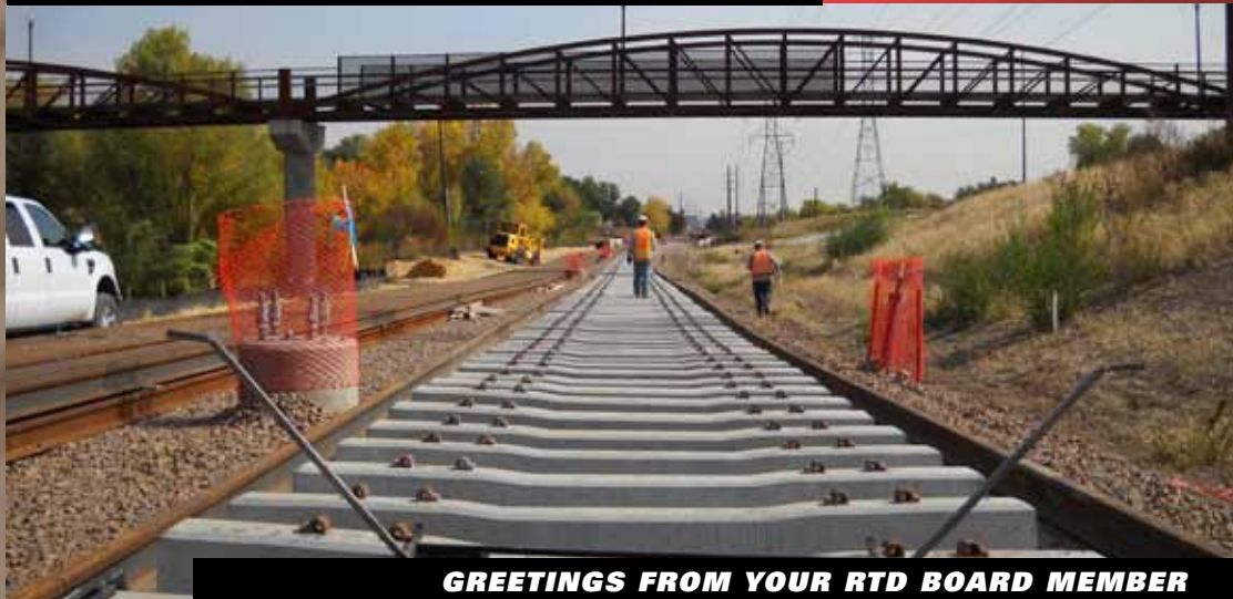
Crews installing light rail track on the West Corridor.
