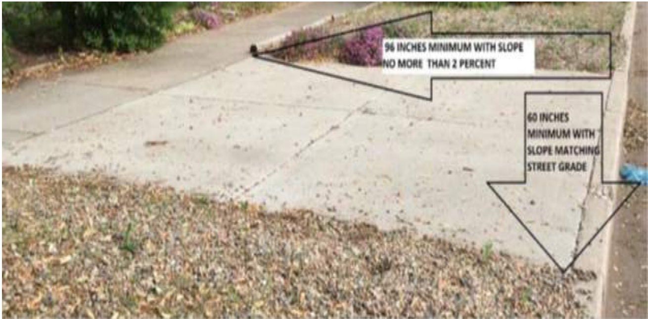
Figure: Bus Pad Dimensions
