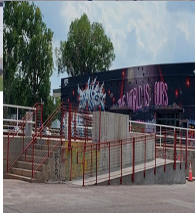
Ramp and entrance behind
