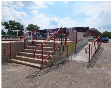
Ramp on N side of building
